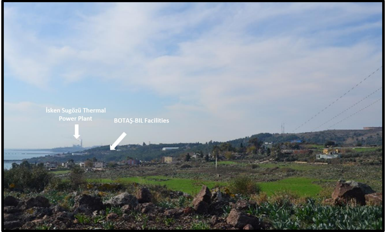
Photo 6: Isken Sugözü Thermal Power Plant (9.7 km to the southwest of the Project Site) and BOTAŞ Facility Premises (1.2 km to the southwest of the Project Site) (view from the Project site)
